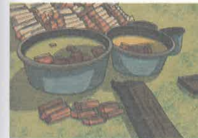
Figure 6.14: Bricks are soaked in water before use
