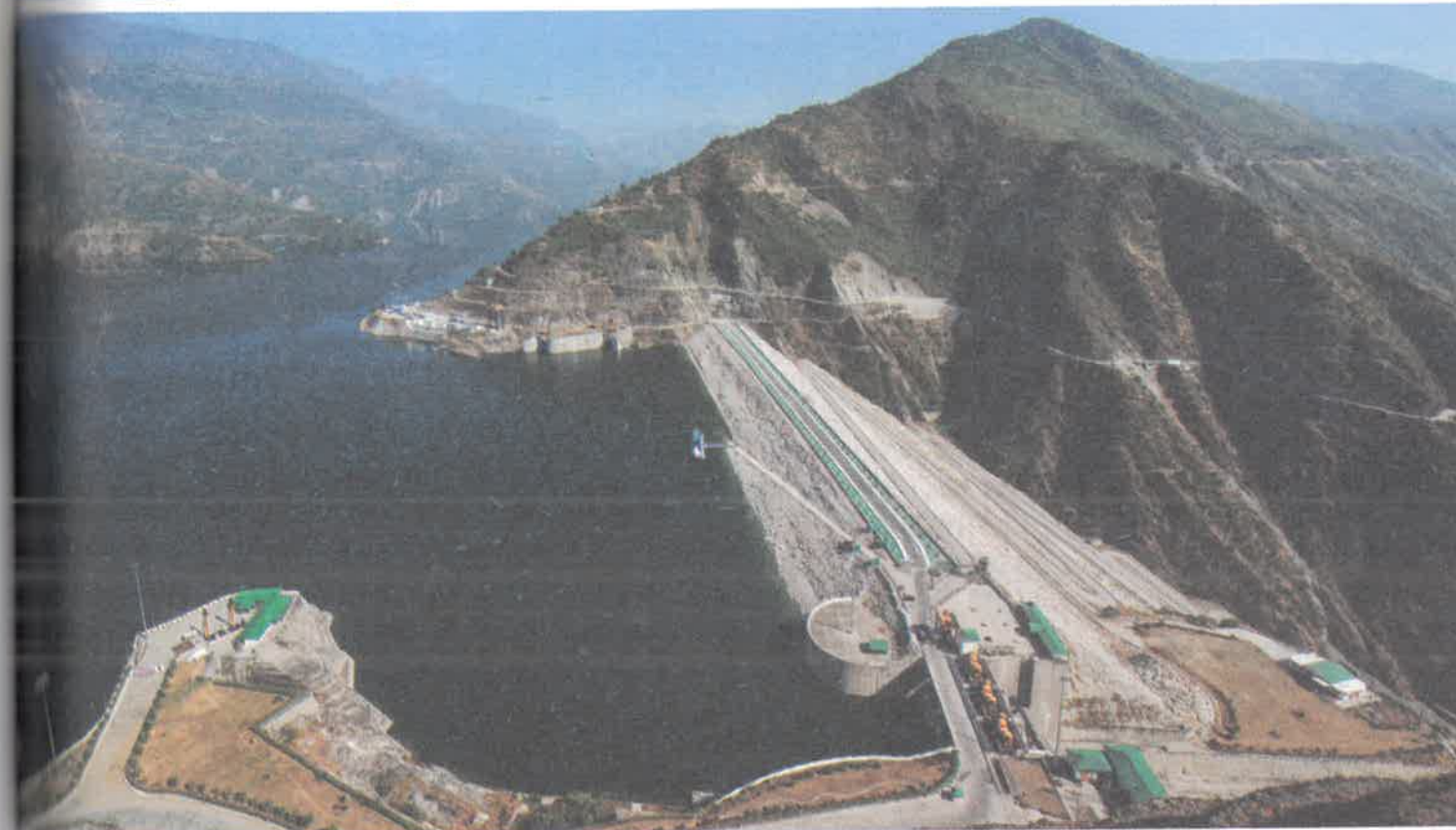
Figure 6.1: Tehri dam in Uttarakhand
