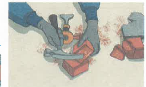
Figure 6.16: Cutting the brick using chisel and hammer
