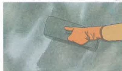
Figure 6.19: Applying plaster on the wall
