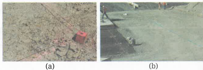
Figure 6.13: (a) Using reference lines for marking site of construction, and (b) marking lines for construction
