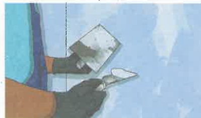
Figure 6.20: Plastering of a wall
